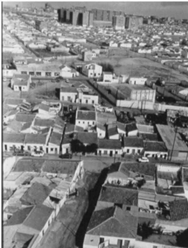
Palomeras before remodeling
