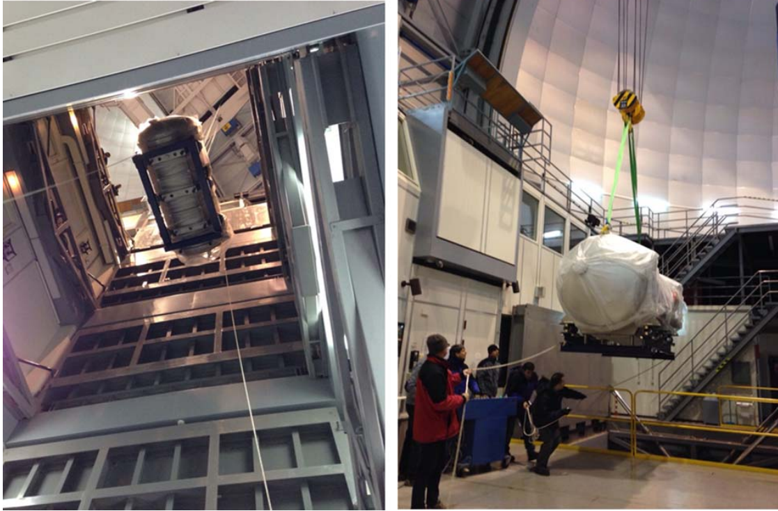
Figure 3. The near-infrared spectrograph of CARMENES was moved to Calar Alto Observatory and installed in the coude laboratory of the 3.5 m telescope on Oct 20, 2015. The vacuum tank of the visible-light spectrograph is very similar; it was installed already in August.
